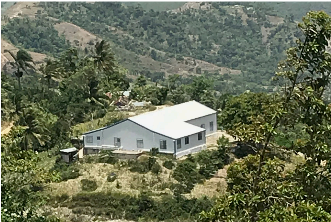
Figure 3. St John's the Evangelist-Petit-Harpon, Haiti, rebuilt after 2010 earthquake, consecrated in 2013.
